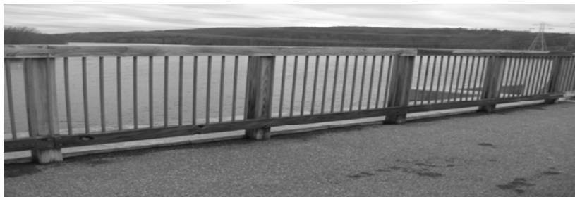
On bridge over Croton watershed
